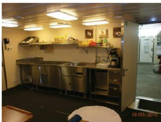
A modern galley with food stores, stove, oven and CO2 extinguishing system.
